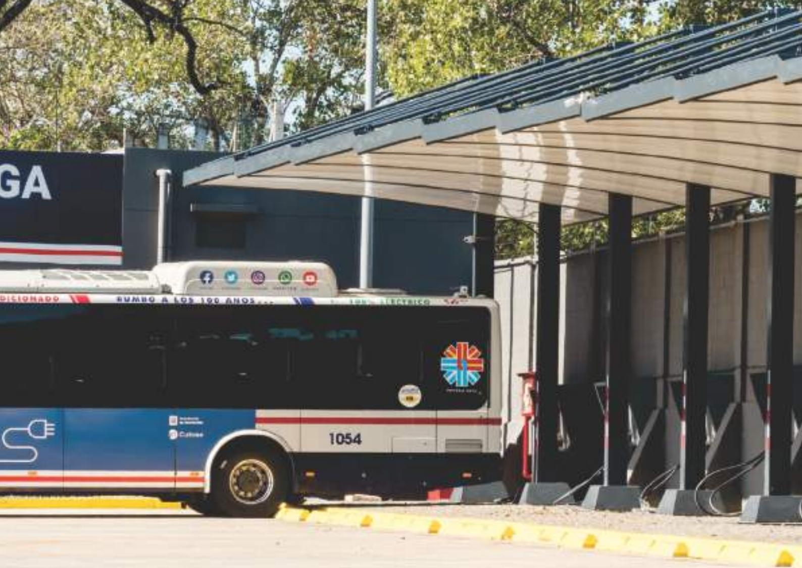
The Charging Center project at the Añón Plant is planned to be able to charge 100 buses simultaneously. In its first stage, 23 BYD chargers are operational, each one with a charging power of 80 kW (40 kW x 2).
